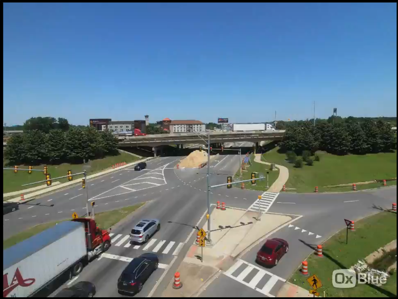
Timelapse of NB Bridge Demolition
