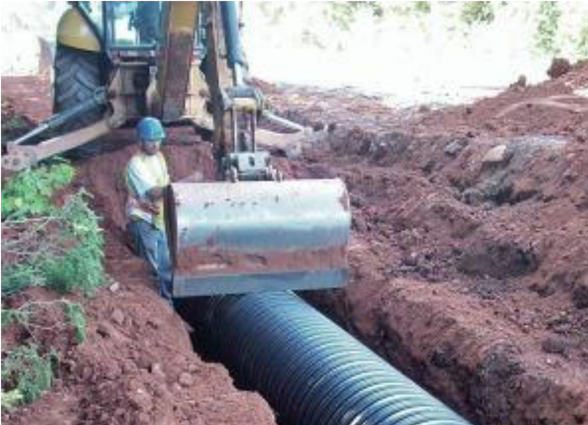
N-12 ST IB SOIL-TIGHT JOINT
