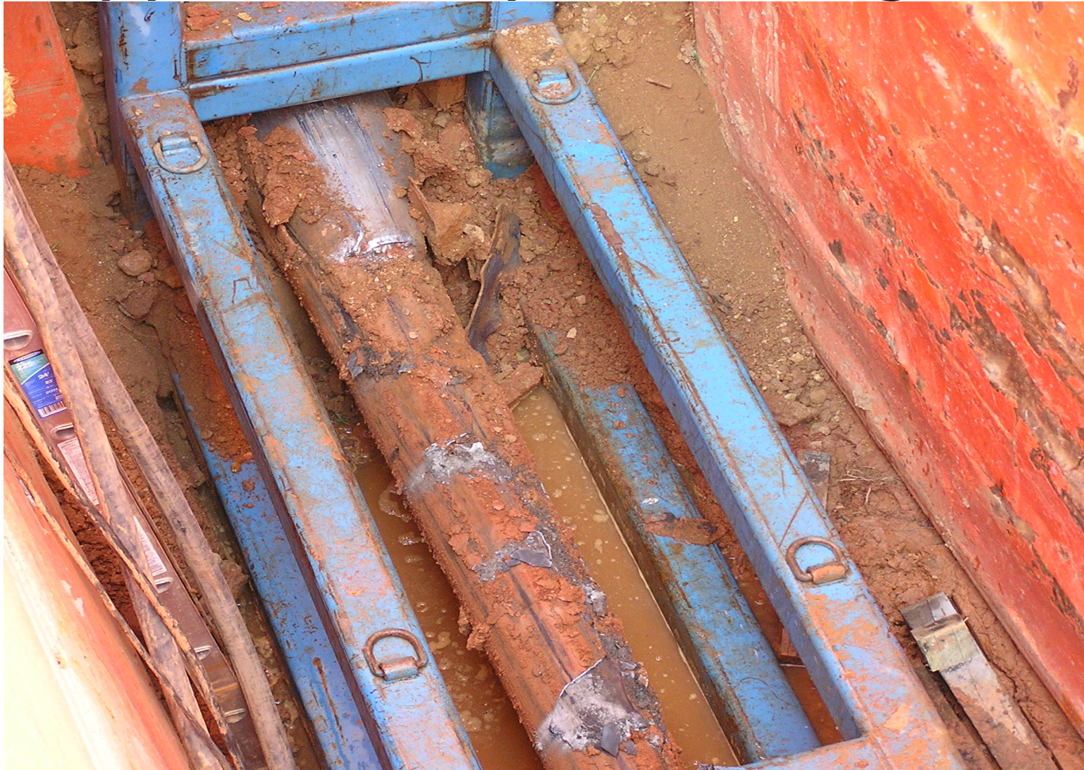
Expander-head Exiting into Pull Pit
