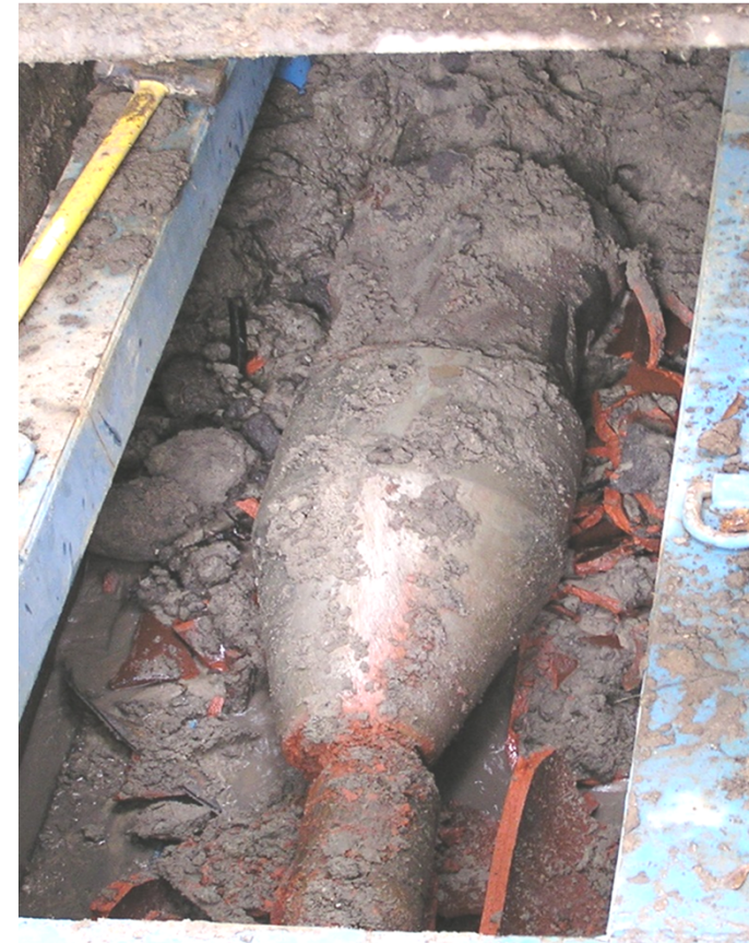
Pipe and Expander exiting pull pit
