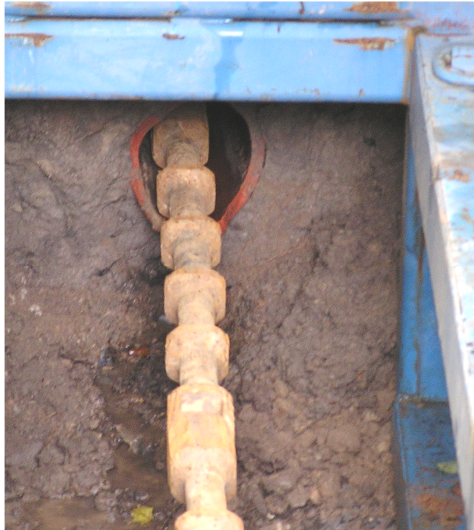
Pull Rods through Clay Pipe
