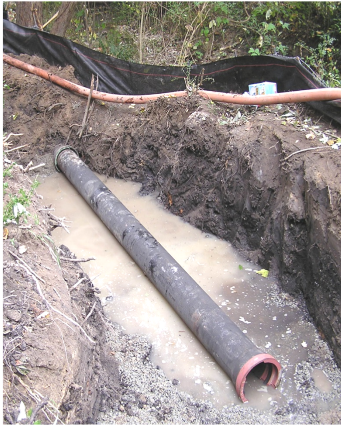
Pipe pulled into expanded Hole-low pulling force Full length pipe keeps prices down
