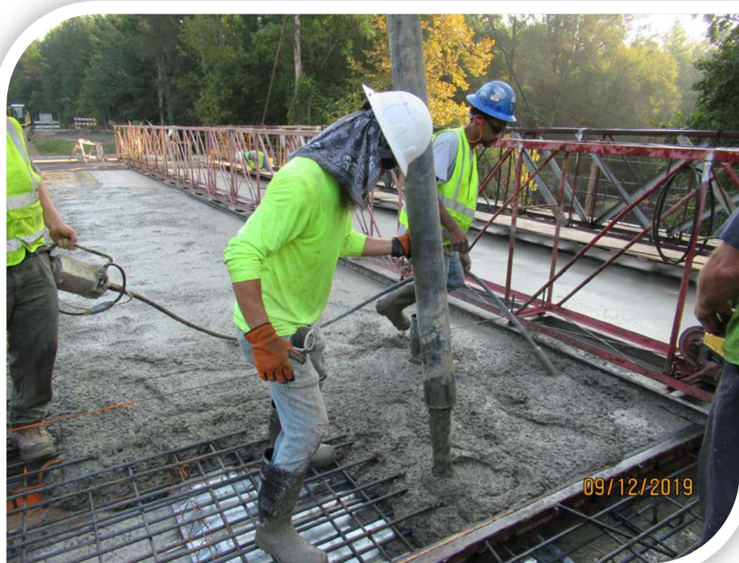
Placement of Concrete Superstructure
