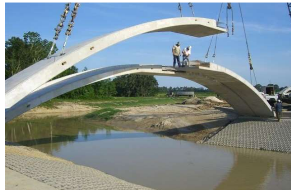
TWIN LEAF CONSTRUCTION
