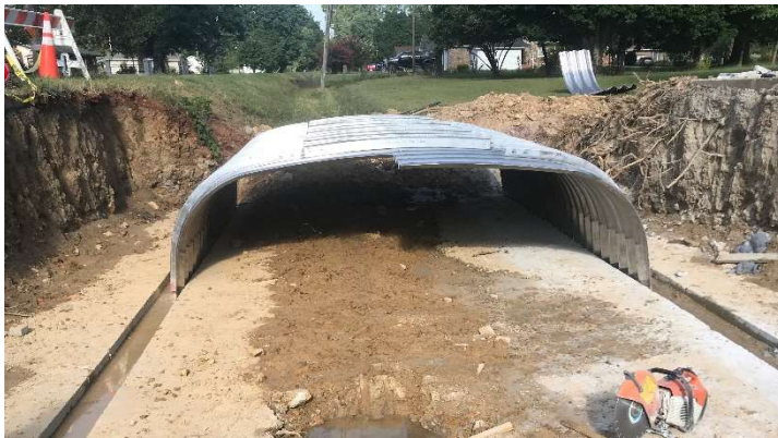
Lift and set in place
